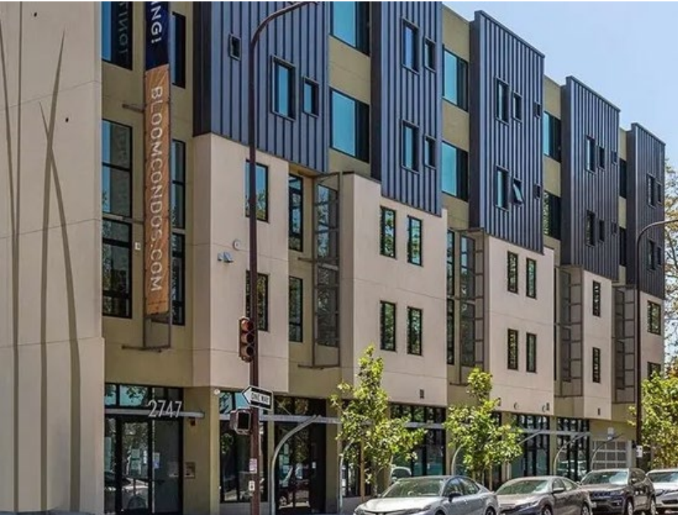
Building Articulation: Façade design and distinct features of building parts
